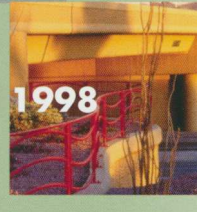
Thunderbird Road Vehicular Bridge Beth Galston
